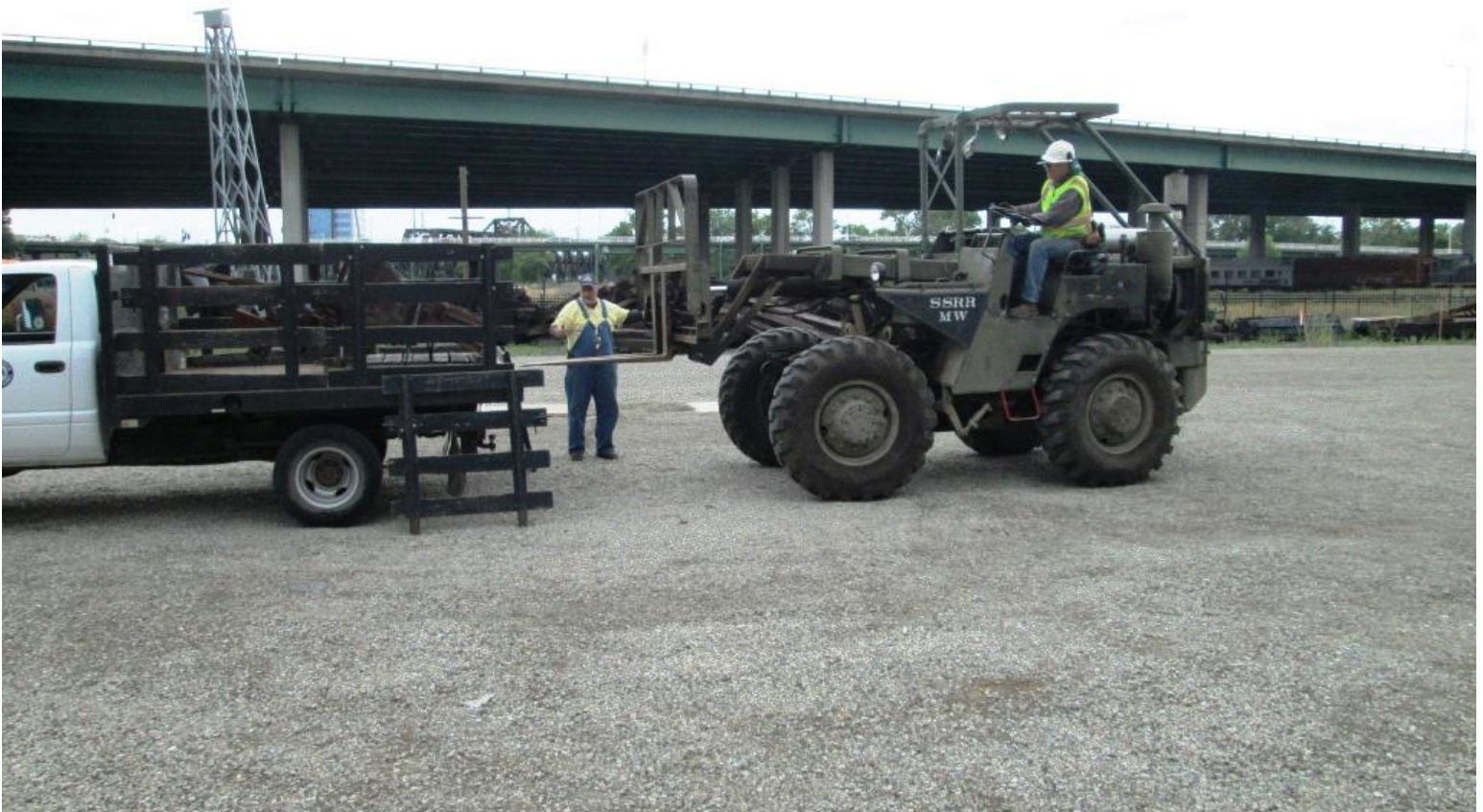
Mike F. guides Steve on our Green Machine to grab the interlocking machine off the truck
