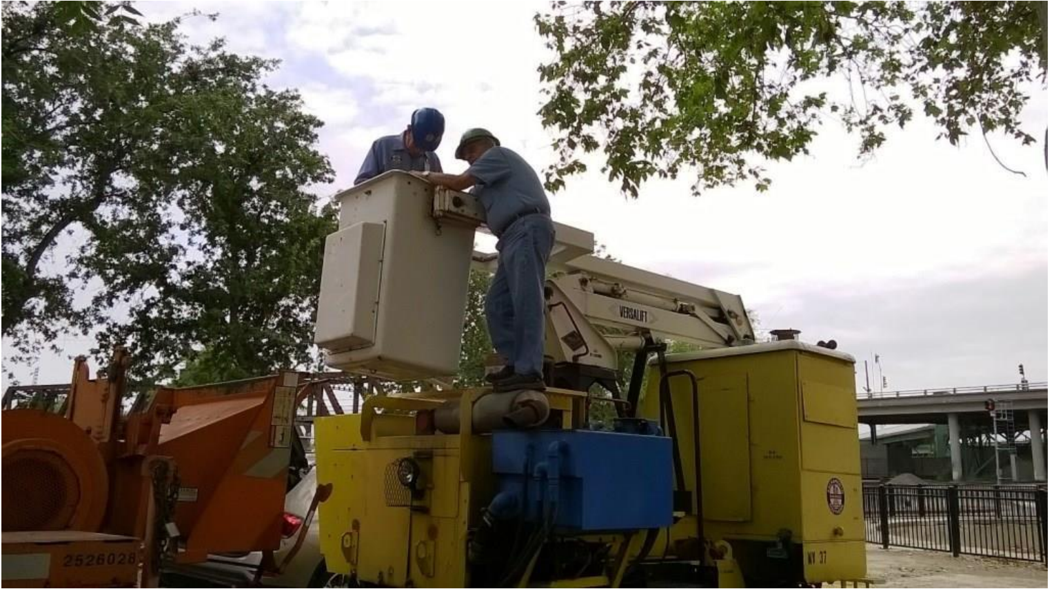
Bill and Dennis repairing the man-lift's bucket control
