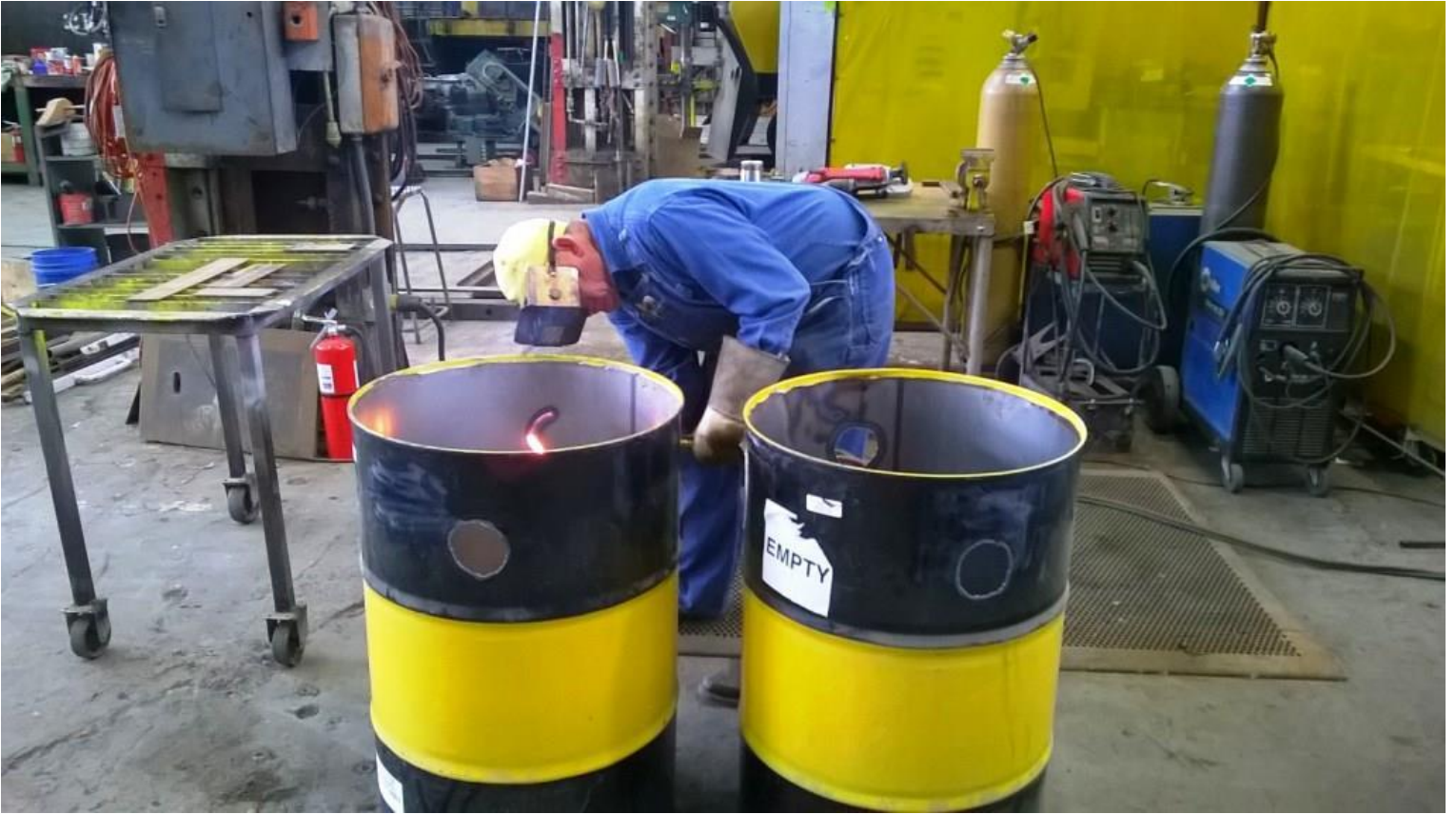
Cliff cuts holes in 55-gallon drums for lifting chains
