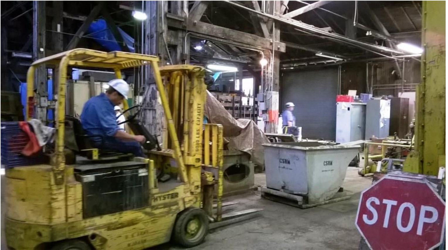
Joe grabs a dumpster to remove it from the bay in the Boiler Shop where roof-work is to commence
