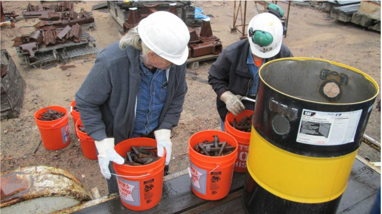
Fred and Heather get buckets of spikes in position for transfer to the 55-gallon drums
